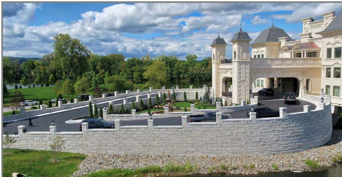
block, three other block types were called out: guardrail block, column block, and capstones. Some wall portions were gravity, other portions were geogrid. The complex design meant a considerable amount of collaboration and communication was needed between the civil engineer, the developer, the manufacturer (Northeast Concrete), ReCon, the wall engineer (Titan), and the wall contractor.
