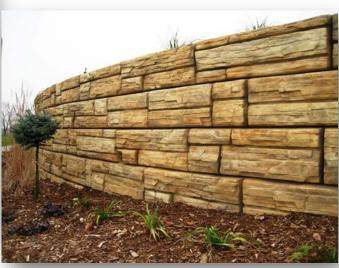
Acid etch stains require an additional degree of care and skill to properly apply. Acid etch stains create deep colors (usually dark browns and rusts) and a natural variation in the color which adds to the authenticity of the finished wall appearance. For additional information on acid etch stains and hybrid stains, please contact ReCon.
