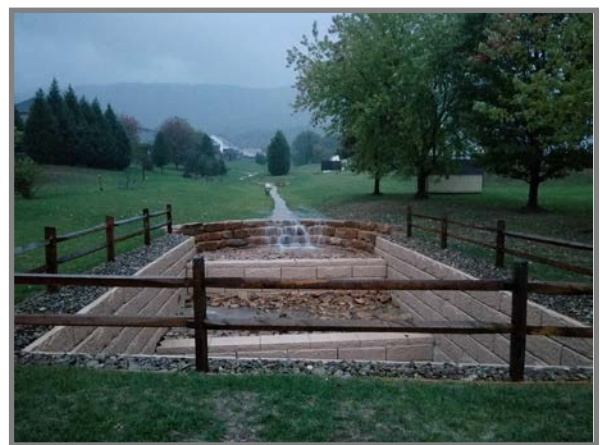
After Improvements, Weirs and Collection Area with ReCon Block.
