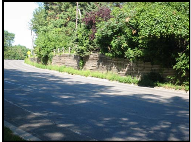
Existing timber wall to be replaced.
